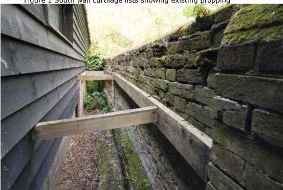
Figure 1 South wall curtilage lists showing existing propping
